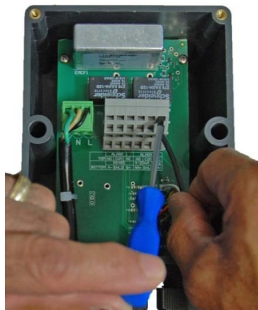
Figure 6: Electrical Connections on Terminal Block (P1)
